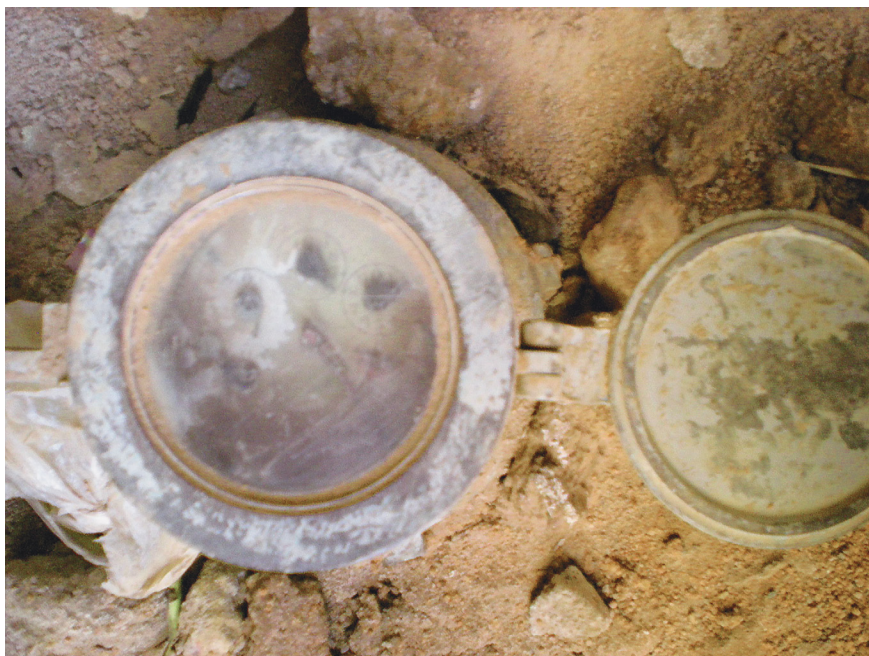
Figure 2. A water meter buried in the courtyard of a house, Deim, Khartoum. L. Arango, 2009
